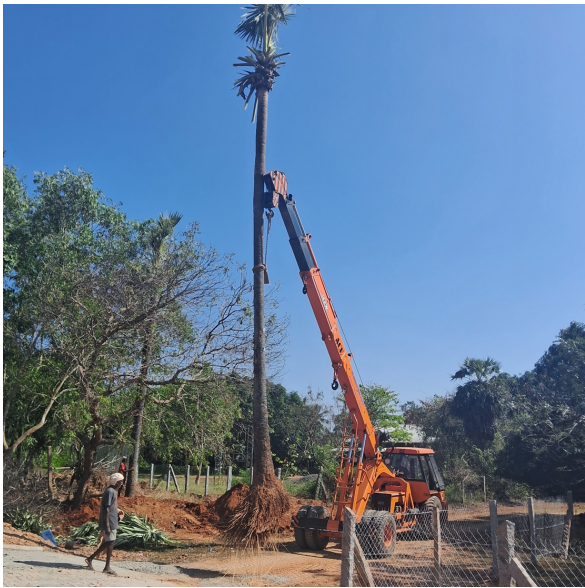
Coordinating planting Palmyra at Radial Road
